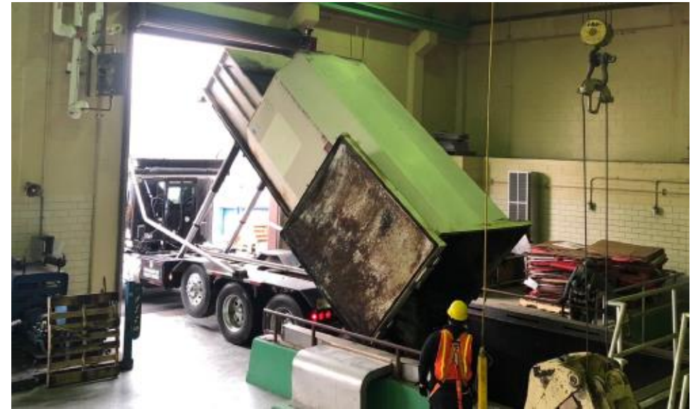
Interior of Tipping Floor
